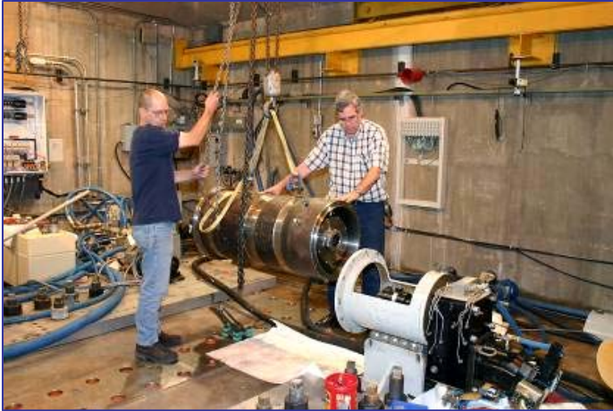
Figure 3. High-speed generator rotor and dummy stator tube during installation
